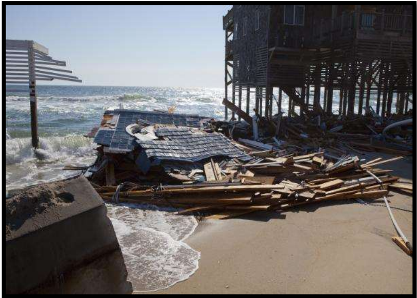
Rodanthe, North Carolina, Sep. 3, 2011. Hurricane Irene destroyed homes and eroded beaches to the point that the waves now reach under this elevated house.
