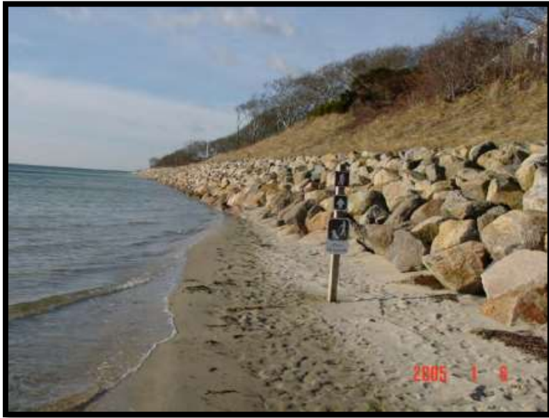
The loss of public lateral beach access due to shoreline armoring along the shore of Chatham, Massachusetts. Prior to revetment construction, a dry sandy beach provided lateral public beach access to a U.S. Fish and Wildlife property. Photo O’Connell, USGS.
