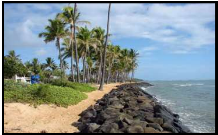
Reduction of beach on Kauai due to armoring. Photo: NOAA
